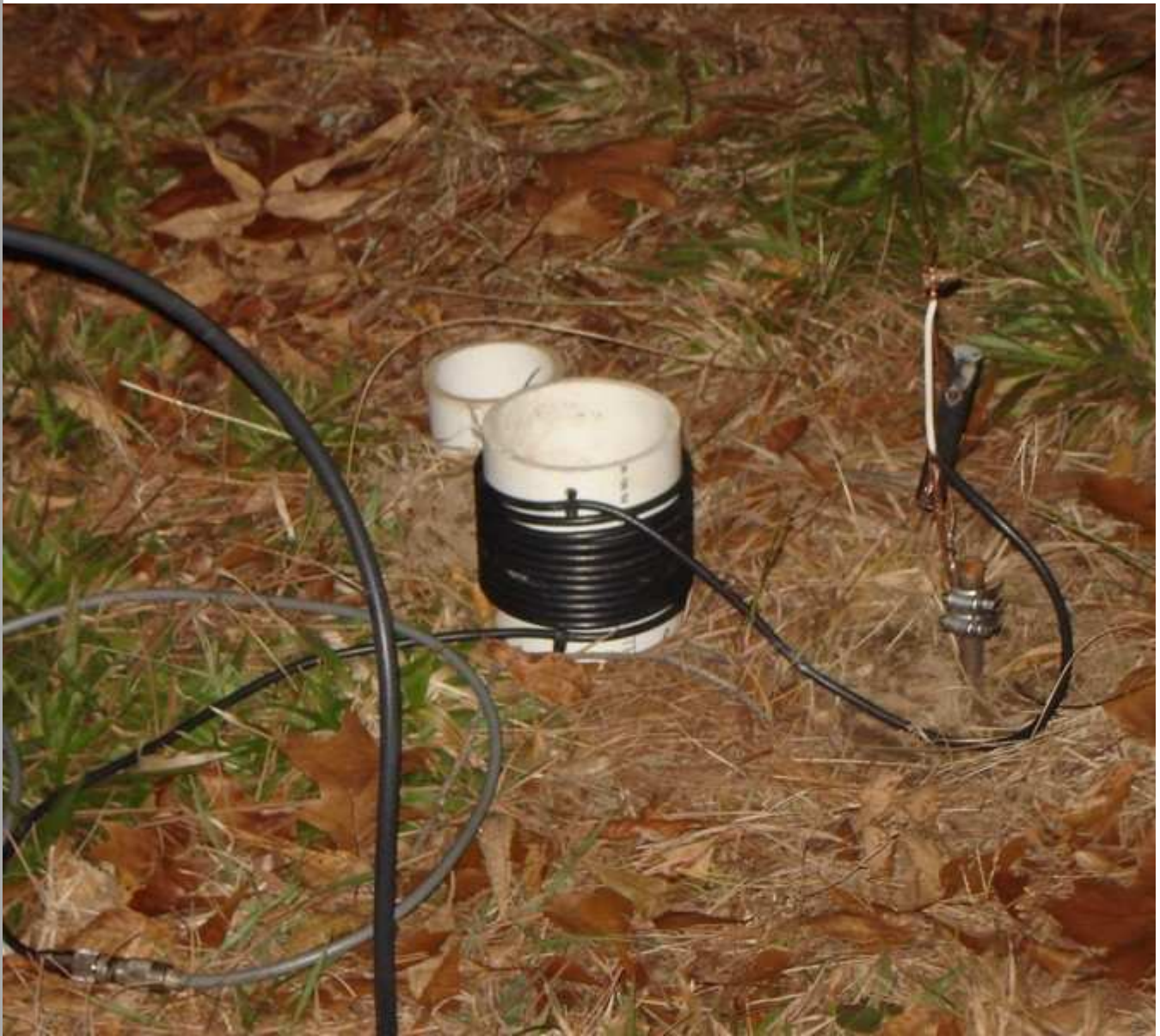
Current Choke, 12 turns RG-8X on 4 inch diameter PVC pipe.
